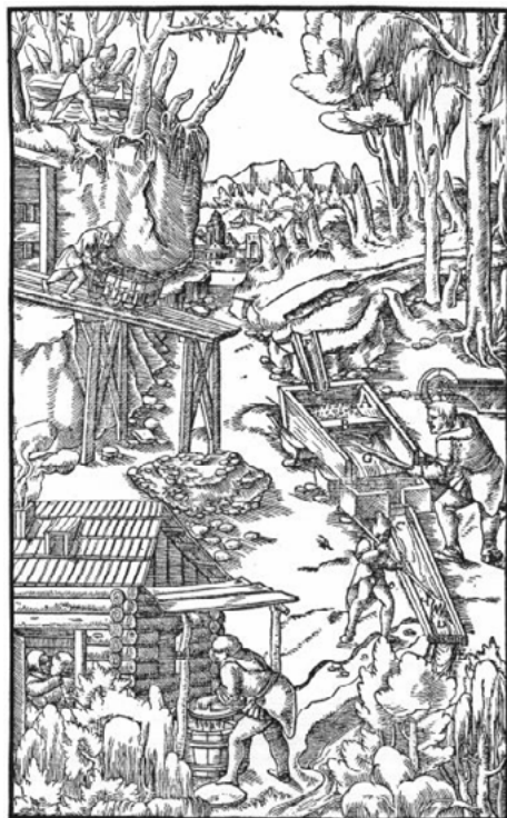
A—BOX. B—PERFORATED PLATE. C—TROUGH. D—CROSS-BOARDS. E—POOL. F—LAUNDER. G—SHOVEL. H—RAIL.
